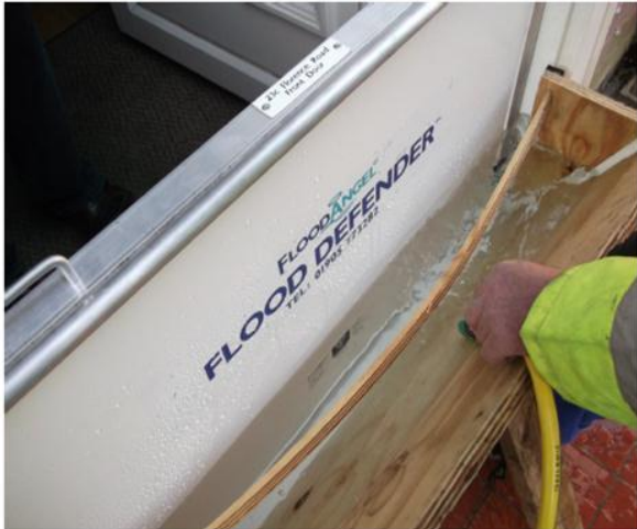
Example of a wet test
